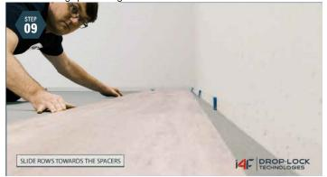
**Use Spacers and Slide Rows Towards Spacers:** Place the spacers along the walls to create an expansion space of 0.2 inches. Proceed by gently sliding rows 1 and 2 towards the spacers.
