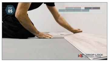
**Align Installation**: Use a full plank (3) as an alignment guide by placing it against the wall. Angle plank 3 into plank 2.
