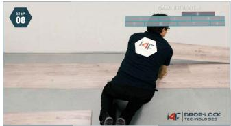
**Remove Alignment Planks:** Remove planks O and 3 by angling them out.
