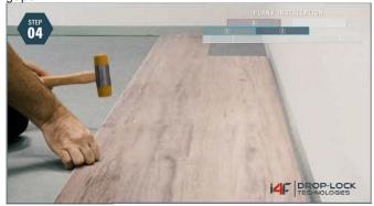
**Engage the Short Sides**: Drop the short side of plank 2 onto the short side of plank 1. Drop & Lock by pushing down firmly, if necessary, use a hard PVC mallet to tap the joints slightly on the short side to secure. This ensures 3-fold locking.
