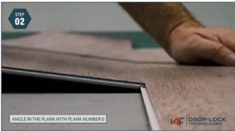
**Align Installation:** Starting from the left with the tongue-side facing the wall, carefully place the first board in place against the wall (plank 0 shown above).
