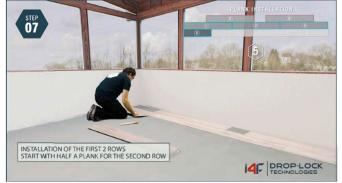
**Finish Rows 1 & 2:** Start your second row by using half a plank (5) and angle in with plank 1. Make sure the short sides are aligned. Repeat the same steps as above to finish the second row. Ensure there are no gaps or height differences.
