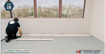
**Finalize Installation:** From row 3 onwards, installation does not require a specific laying pattern. To finish the last row, measure the distance from the wall to the last installed row minus 0.2 inches. Remove spacers when installation is complete. Finish up the room by placing any plinths, molding and trim.
