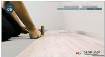
**Install Plank 4:** Take another full-length plank and angle it into plank 3. Then slide plank 4 until the short side contacts the short side of plank 2. Drop & Lock by pushing the planks firmly down, if necessary, use a hard PVC mallet to tap the joints slightly on the short side to secure. Ensure there are no gaps or height differences.
