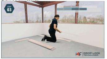
**Install Plank 2**: Take another full length plank and angle it into plank 0. Then slide plank 2 until the short side makes contact with the short side of plank 1.
