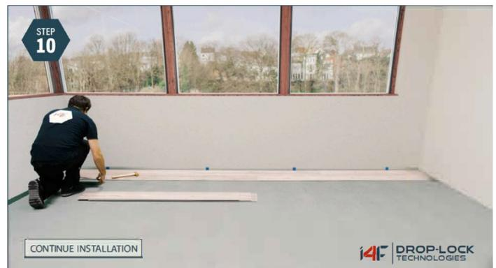
**Finalize Installation:** From row 3 onwards, installation does not require a specific laying pattern. To finish the last row, measure the distance from the wall to the last installed row minus 0.2 inches. Remove spacers when installation is complete. Finish up the room by placing any plinths, molding and trim.
