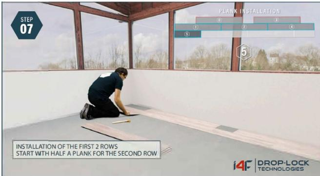
**Finish Rows 1 & 2:** Start your second row by using half a plank (5) and angle in with plank 1. Make sure the short sides are aligned. Repeat the same steps as above to finish the second row. Ensure there are no gaps or height differences.
