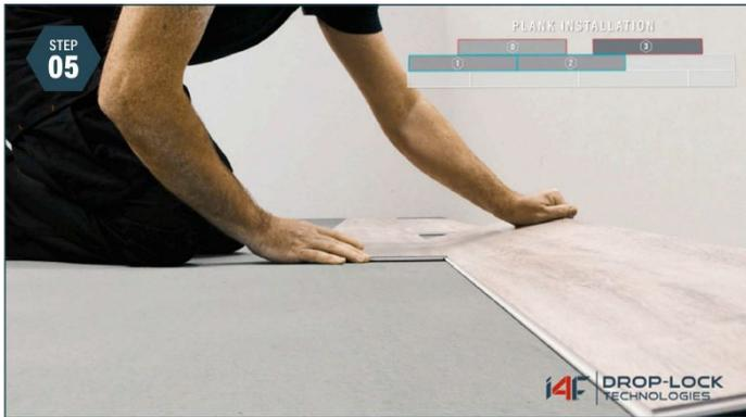
**Align Installation:** Use a full plank (3) as an alignment guide by placing it against the wall. Angle plank 3 into plank 2.
