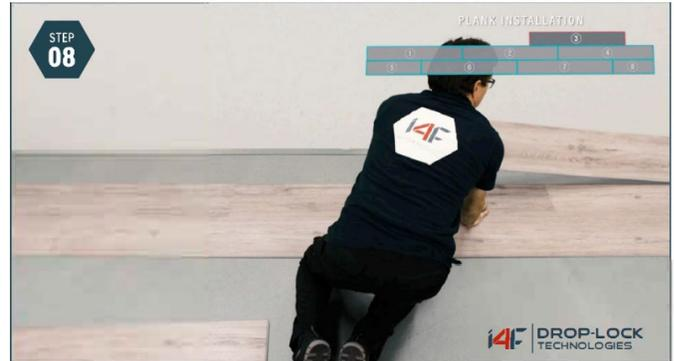
**Remove Alignment Planks:** Remove planks 0 and 3 by angling them out.
